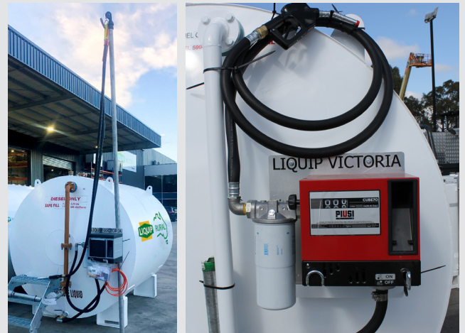
Liquip Rural Farm Tank and Solar Fuel Dispensing System
